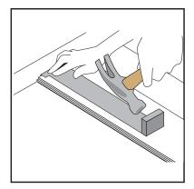
After engaging the side joints in the last row, slightly lift the edge of the plank. Using a pull tool, pull the plank completely into place. Follow up the length of the plank a second time and tap to ensure the joint is completely locked.
