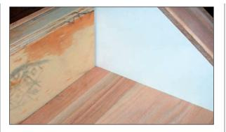
Step 8: Dry-fit the treads and risers. Never force a tread or riser into place. Trim as necessary. Back-cut a slight angle on the riser ends approximately ¼ inch behind the face to prevent the riser from snagging the drywall and provide a better fit.
