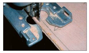
• **Step 5:** Use these measurements to cut the tread and riser for the first step. Accuracy is crucial. Miter saws don't cut the closest, and jigsaws can rip out a lot of material, so first use a jigsaw to cut as close to the scribe line as possible.
