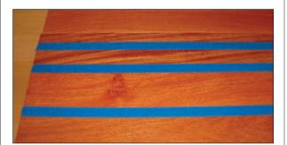
• **Step 1:** Latex paints can be applied over a floor with at least two coats of well dried surface finish or over any factory-finished product. Using a long-lasting, easy-release tape, lay out and tape off the design, making sure the tape is properly secured by rubbing the edges. Lightly sand the areas to be painted with 120-grit or higher sandpaper, making sure the finish powders lightly. As you sand, slightly overlap onto the tape.
