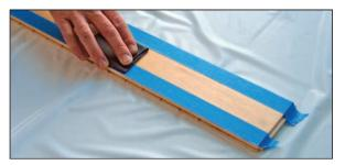
• **Step 2:** Once the floor is taped off, it must be abraded. Use a grit of at least 200; here the board is being abraded with 320. If you're doing a large area, you can use a buffer and a maroon pad. Abrading the floor helps the tints stick to the floor and also heats up the tape, creating a better bond at the edges. After abrading, tack the floor with a slightly wet cloth.
