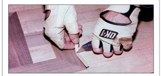
• **Step 1:** Use a razor knife to cut the sliver to the necessary length.
