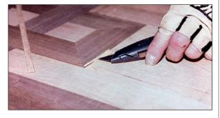
• **Step 5:** With the sliver down as far as it will go, use the razor knife to score both sides of the sliver at the floor line, slicing off the excess.
