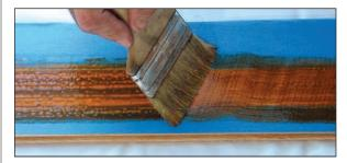
Step 6: Next, immediately go over the same area, but this time, slightly jiggle the brush back and forth as you go down the board, creating the look of grain. To soften the effect, just barely touch the tint in a back-and-forth motion with a makeup brush.
