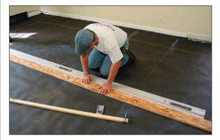
Install a minimum of three rows against a straight-edge, starter board or backer board attached to the floor along the working line.
