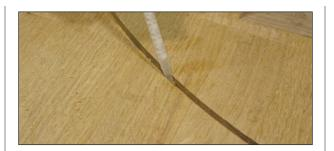
Apply adhesive into the channel. Do a section at a time, since most epoxies have only a five-minute working time. Place the metal into the channel and install nails into the predrilled holes before the adhesive cures.
