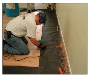
When installing prefinished product, the surface should be protected from scratches by applying tape or another protective surface on the face of the base plate of the cutting tool. Cutting prefinished products may require easy-release tape along the cutting line to protect the surface, prevent chipping and to eliminate edge burring.
