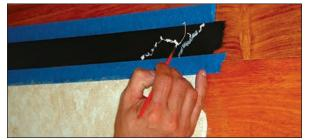
• **Step 5:** Use a small brush to hand-paint the vein effect of the desired marble.
