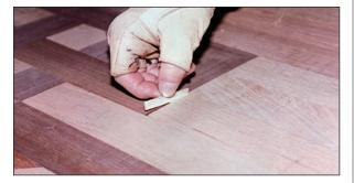
• **Step 3:** Insert the sliver with the narrow side down. If the gap is too narrow for the sliver to go in deep enough, a razor knife can be used to slightly expand the gap.
