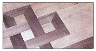
• **Step 7:** Allow the glue to set before sanding the floor.
