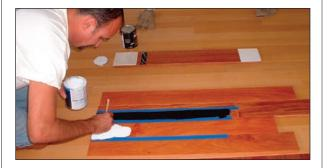
• **Step 2:** Vacuum and tack the area of the design and the surrounding areas. Paint the latex base coats according to your drawings. Remove the tape while the paint is still wet. Then, allow the paint to dry thoroughly (a minimum of 24 hours or more depending on job-site conditions).
