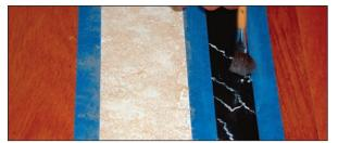
• **Step 6:** With a slightly bigger brush, smooth the veining while it is still wet, working in all directions and pushing down until the paint matches the sample.
