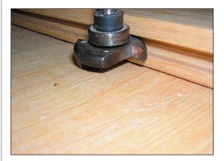
• Prior to installing the border, cut a groove for a slip-tongue or spline where necessary, using a router bit designed for the thickness of flooring.
