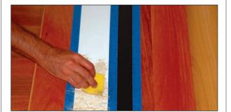
• **Step 3:** Re-tape the borders, securing the tape well. Then, for the stone effect, use the appropriate sponge, applying the texture to match the approved sample.
