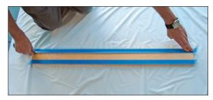
• **Step 1:** Use easy-release tape to carefully mark off the areas to be painted, and roll the tape to ensure a good bond at the edges.
