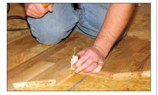
• Use a sharp chisel or corner chisel to clean up areas, such as corners, not removed by the router
