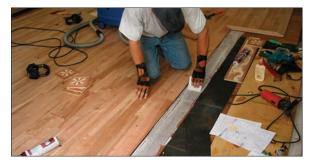
Following the border manufacturer's instructions, spread the approved adhesive onto the subfloor. Use the trowel size and profile recommended by the adhesive manufacturer and heed the flash-time and open-time directions.
