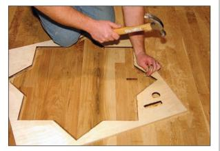
If you expose nails on any pass, use a nail set to drive the nail further into the floor and out of the way of the router bit.
