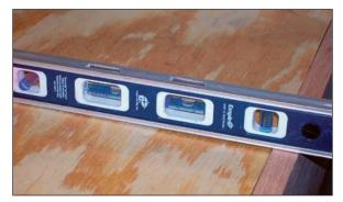
• **Step 2:** Use a level to check the rough tread for flatness and the rough riser for plumb. Shim if necessary to make the angles between the tread and riser 90 degrees.
