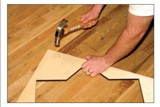
• Fasten the template to the field flooring. The template can be fastened with double-sided tape, or by finish nailing into the field flooring between the floor boards.
