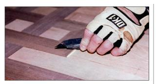
• **Step 4:** The knife can then be used to tap the sliver down. To withstand several sandings and have holding power in the floor, most of the sliver should go down into the gap.
