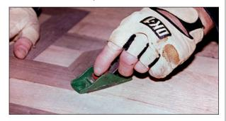
• **Step 6:** To smooth the sliver perfectly even with the rest of the floor, you can use either a small block plane or a sharp hand-scraper.
