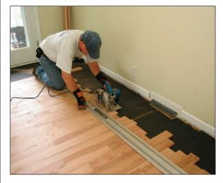
• Resquare your field and cut the field flooring back to the border working line. Use a straight-edge as a guide to cut the ends of the field flooring along the border line.
