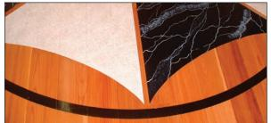
• **Step 7:** After the paint is completely dry, finish the floor with a minimum of two or three coats. Always use the same finish that was used on the original coats (for prefinished flooring, check with the flooring manufacturer for finish compatibility). As an added detail, different sheen levels can be used on different textures and finishes.
