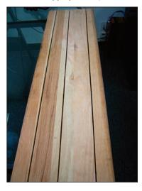
• **Step 9:** Kerf the bottom of each tread lengthwise approximately one-third into its thickness. The kerf channel reduces the tension placed on the stair, helps with adhesion and helps prevent cupping.
