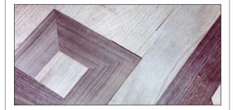
The best way to disguise a gap between boards such as the one against the French knot above is to use the slivering technique.
